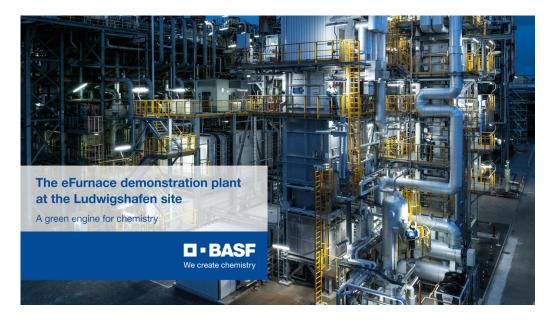
In the eFurnace demonstration plant, two heating concepts are being tested in parallel: direct heating, where the electric current is directly supplied to the process pipes inside the reactor, and indirect heating, using radiant heat from heating elements surrounding the pipes.
